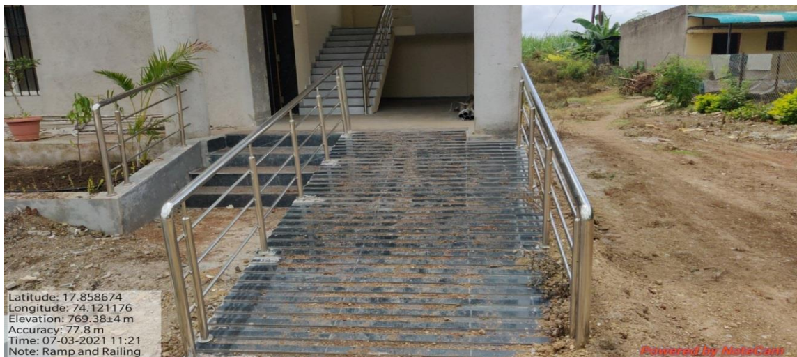
Fig. 2 Ramps & Railing at the entry of the College
