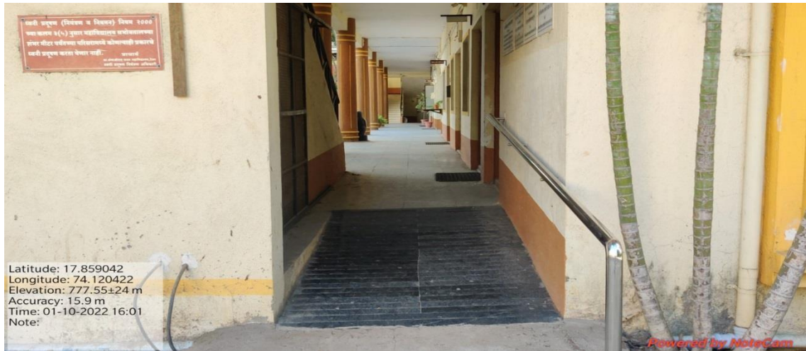
Fig. 1 Ramps & Railing at the entry of the College
