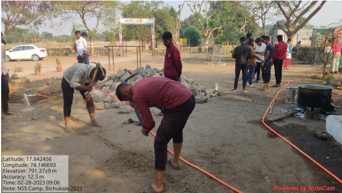
Rain Water Harvesting Project in the College at Bichukale Date: 28.02.2023
