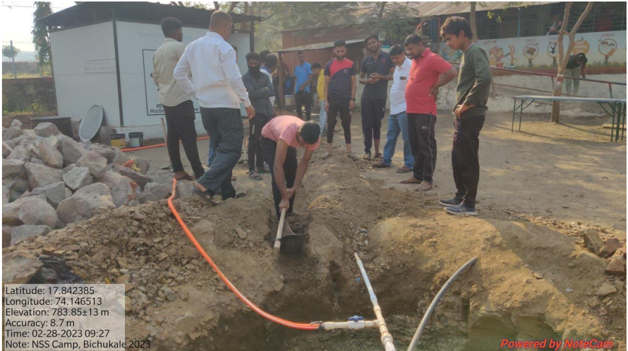
The Roof Water Harvesting and Bore well recharge project A Collaboration Activity with: Gramnachayat Bichukale, Tal. Koregaon Dist. Satara
