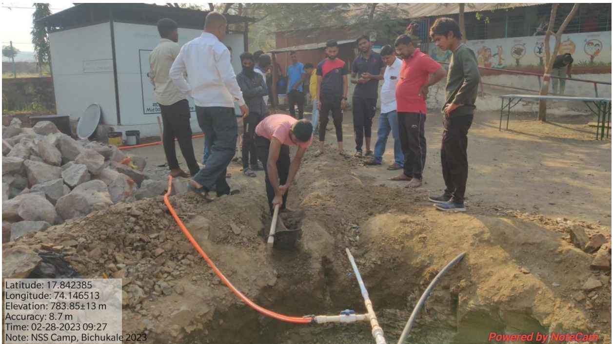
The Roof Water Harvesting and Bore well recharge project A Collaboration Activity with: Gramnachayat Bichukale, Tal. Koregaon Dist. Satara
